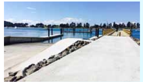
The cement boat launch with floating pontoons on each side, allowing for safer boarding.
