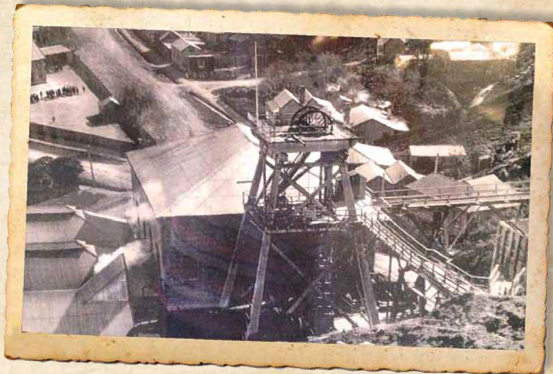
The tall scaffolding, called a poppet, may well once again dominate the skyline of Thames. Help the Society to rebuild this Poppet Head on its original site at the Bella Street Pump House.
